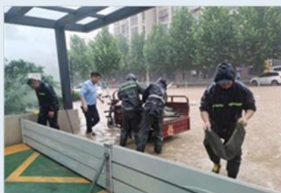
Property administrators raise the flood control wall
